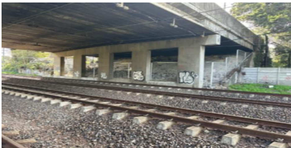
Kindroggen Flats/Masonic Temple Security upgrade:
